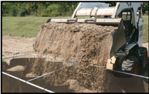
Geocells can be filled manually or with standard construction equipment
